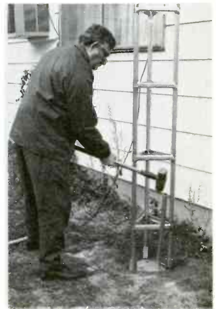
Fig. 11 To prevent the tower from tipping, the base plate is firmly secured by three base stubs, which are driven into the ground.
