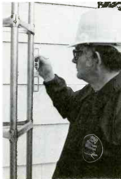
Fig. 10 Gentle taps of a sledge hammer moved the bottom of the tower to provide true vertical, as measured with a level.
