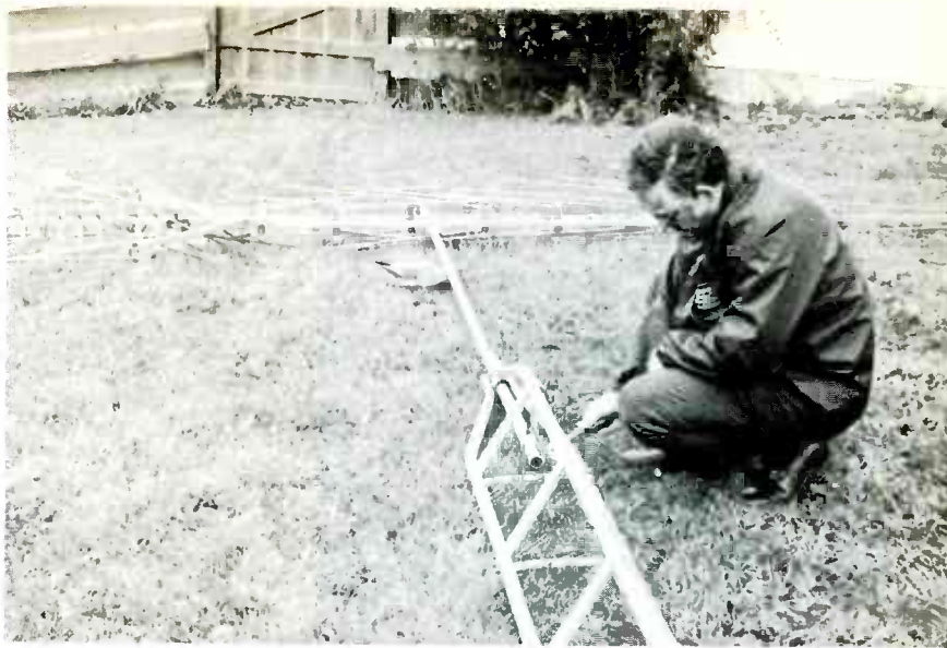
Fig. 4 The mast, preamplifier, and antenna are assembled and attached to the tower.
