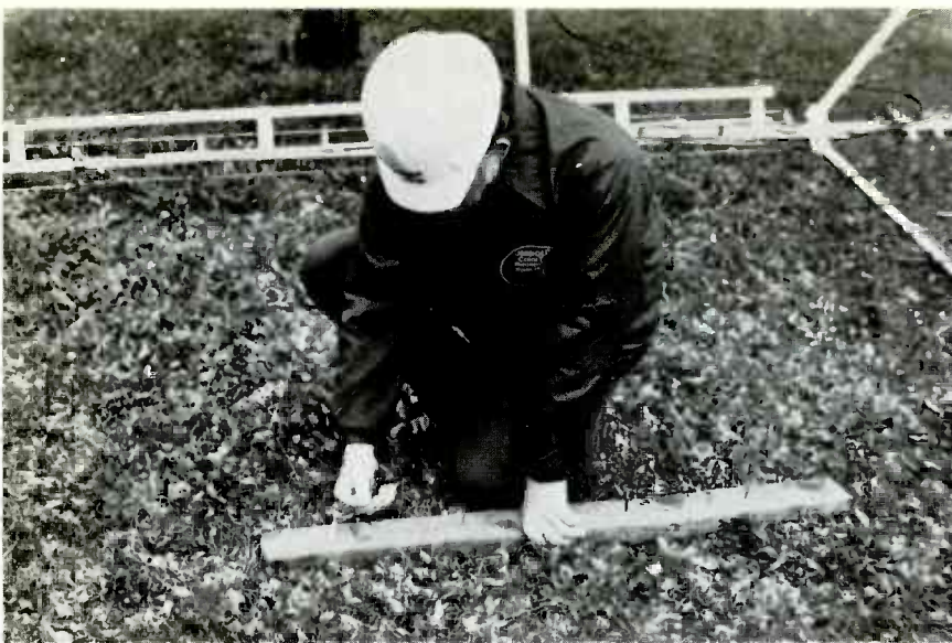
Fig. 6 Prepare the 2X4 with nails and lag screws for mounting under the eaves.
