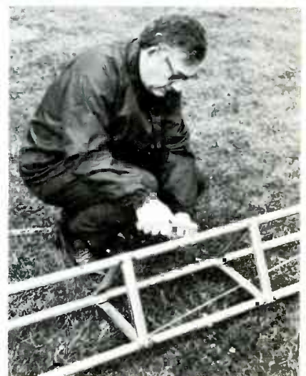
Fig. 2 Various sections of the tower should be assembled on the ground.
