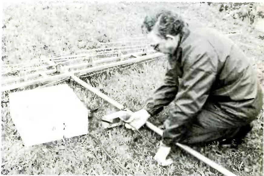
Fig. 5 Coax cable is not sensitive to metal near it, so standoffs are not necessary. However, the coax should be secured, perhaps by layers of plastic tape, to the mast and the tower, thus preventing it from being moved by the wind.
